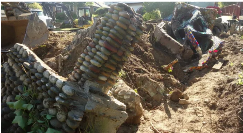
Going, gone... the demolition, June 2, 2021. Photos by Eric Scigliano unless otherwise noted.
